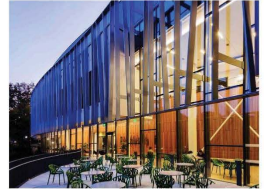
Metallic screens on the facade of Ennead's Bridge for Laboratory Sciences at Vassar College warn birds of danger. © RICHARD BARNES
