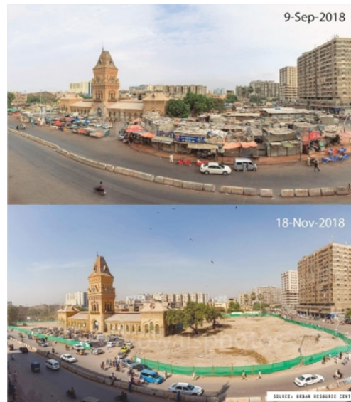
Before and after demolition of 'encroachments'
