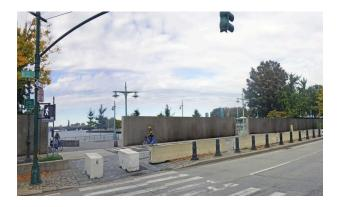
**Proposed USACE Floodwall in Manhattan,** NY Source: Army Corps of Engineers
